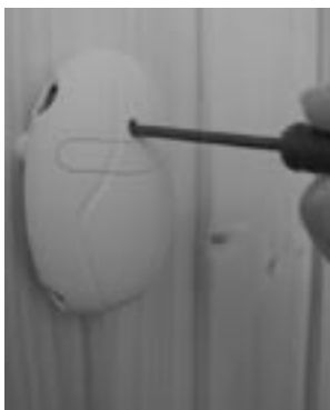
Figure 32. Reset button for overheating limiter
